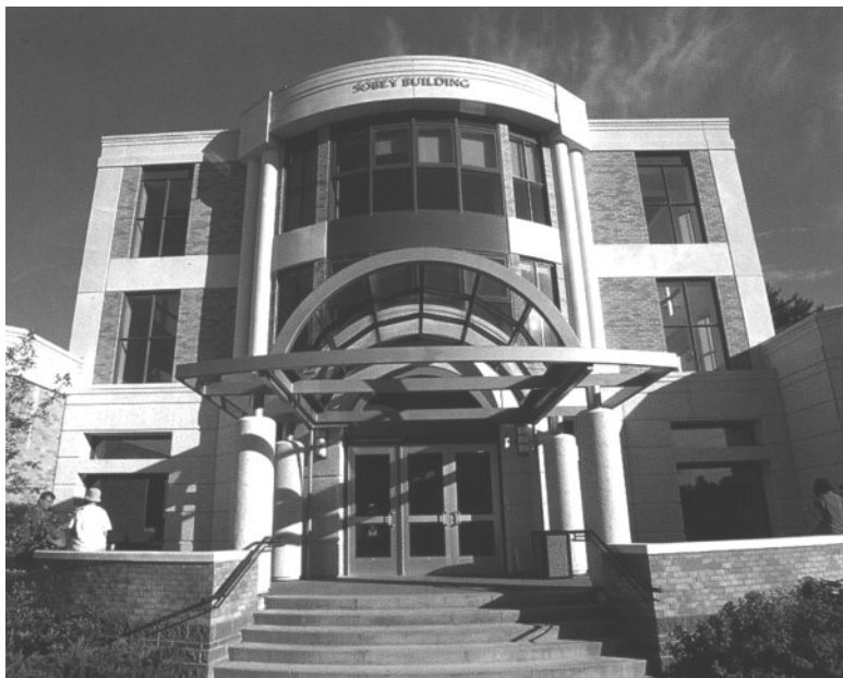
The Sobeys Building housing the Sobeys School of Business.
